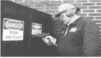
Test switchgear, transformers, vb. for arcing, tracking & corona.
